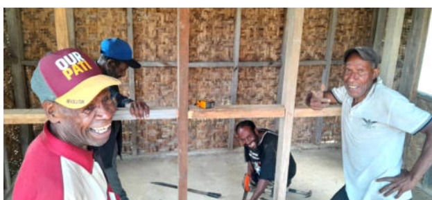
Small clinic under construction.
