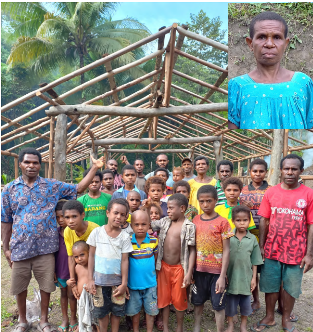
A new place of worship being erected in Monica Paul's village.
