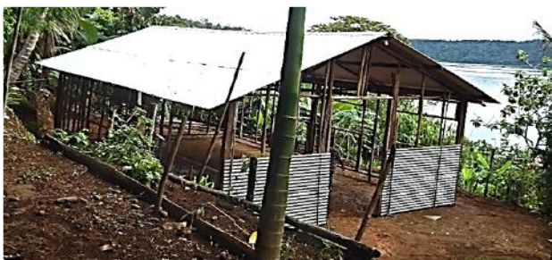
Yombo Island Church with a new roof.
